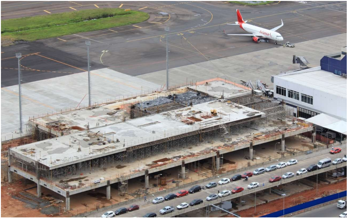
Passenger Terminal Enlargement
