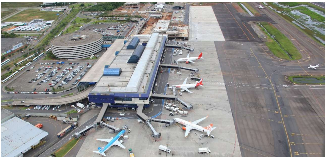
Passenger Terminal with enlargements constructions
